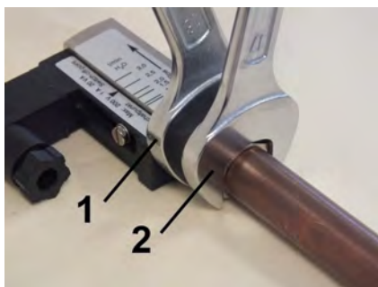
Fig. 10: Screw in the device
