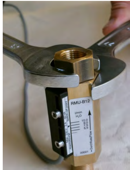
Fig. 35: Tighten process connection (outlet)
