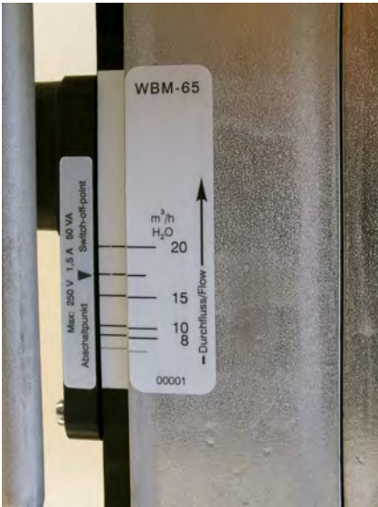
Fig. 34: Reading-off the switch point value (Example)
