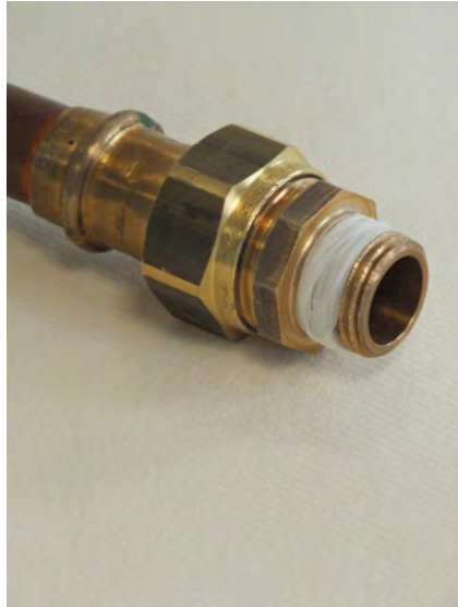
Fig. 11: Pipe connection with sealing thread
